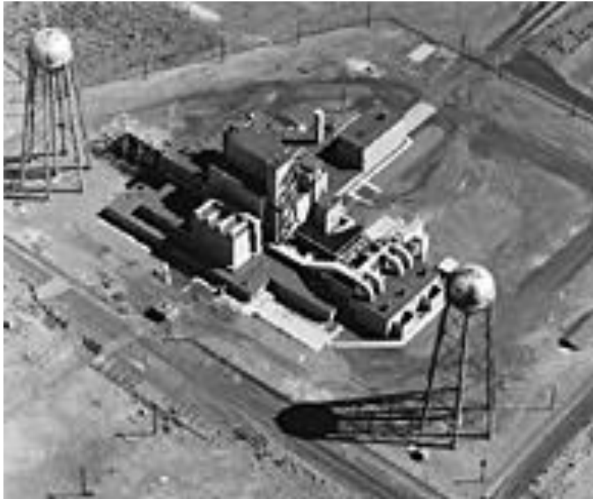
C Reactor Interim Safe Storage at Hanford
