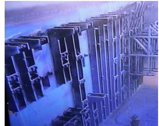
Spraying fixative at the PFP/PRF and “Fixed” Contamination in Blue
